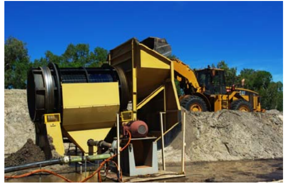
Loader feeding ore into the new In-pit Slurry Unit
