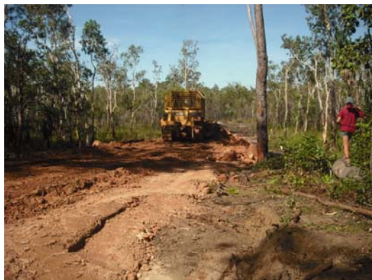
Clearing the road into Lethbridge South
