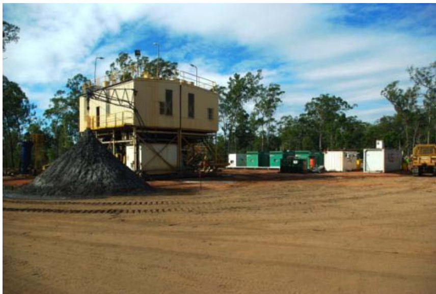
First concentrate production from the Lethbridge processing plant.
